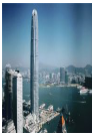
415 metros 2003 Hong Kong (Hong Kong) China, Asia Arq. César Pelli
